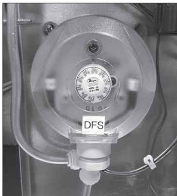
FIGURE 22.2 - DIRTY FILTER PRESSURE SWITCH
