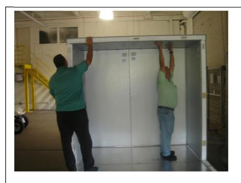
6- Finish corner by installing ceiling panel, and continue assembling in floor / wall / ceiling in "rings."
